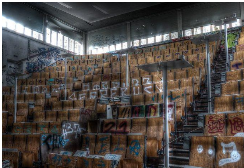
Abandoned University Institute for Anatomy, Berlin. Source: https://ucuccommons.org/2021/05/19/creating-cracks-for-collective-care-in-the-ruins-of-the-university/
